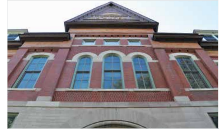
The International Union of Bricklayers & Allied Craftworkers awarded the 2017 Best Comprehensive Restoration Project award to the Bricklayers and Allied Craftworkers Local 8 of Illinois for its work on the Natural History Building. ■
